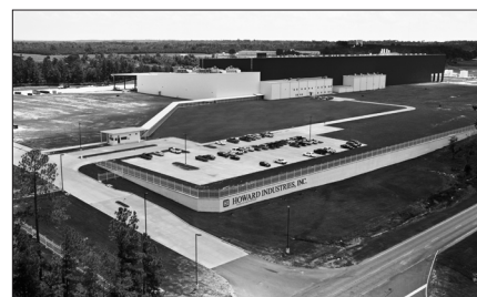
Figure 2: Howard Industries Substation Plant, Ellisville, MS
